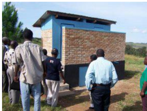
Fig.2 OSIENALA team inspecting an Ecosan Toilet constructed in a school
