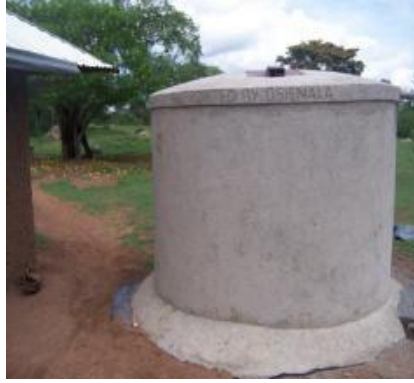
Fig.1 A ferro-cement tank constructed in a home in Kajulu
