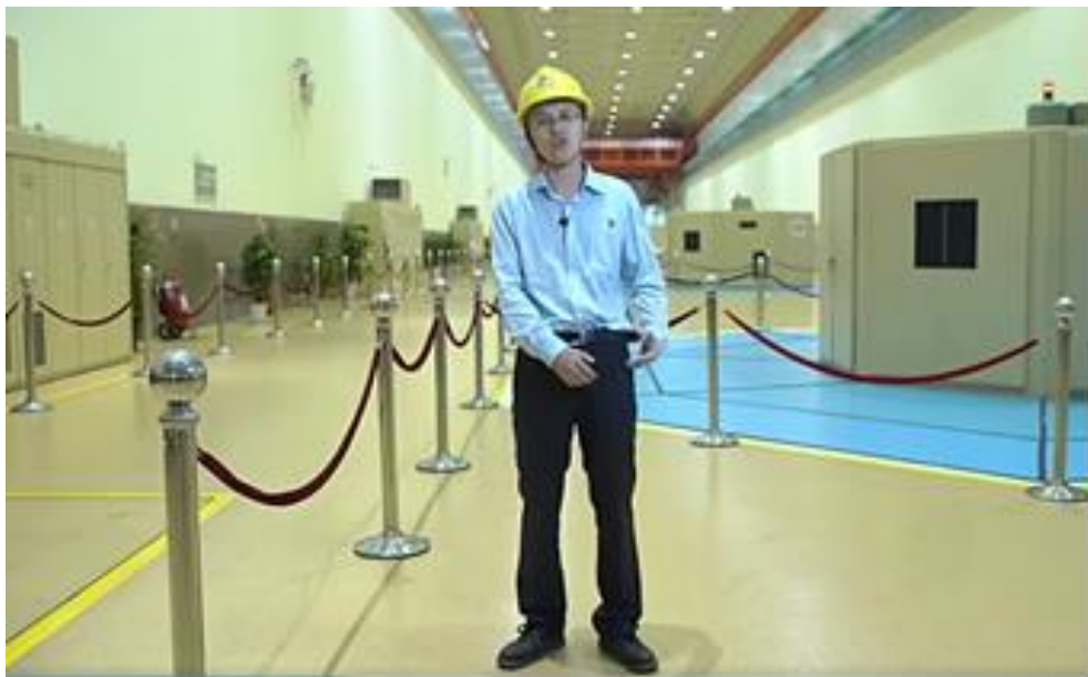
Online Visit to Tianhuangping Pumped-Storage Hydro Plant
