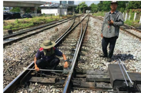
Test at Bangsue Locomotive Depot, Switch No.9B “๙๙9”
