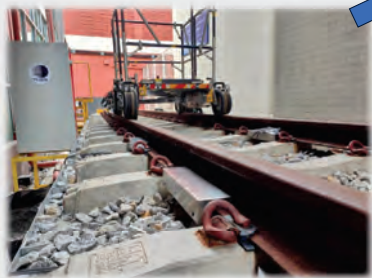
TWD install on the track
