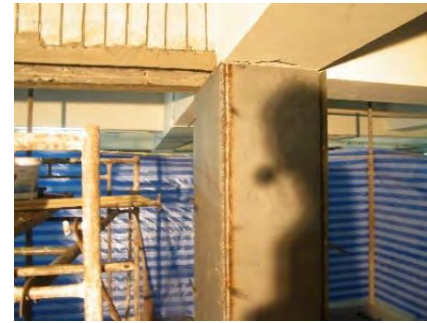
Steel jacking by steel plate and steel encasement.
