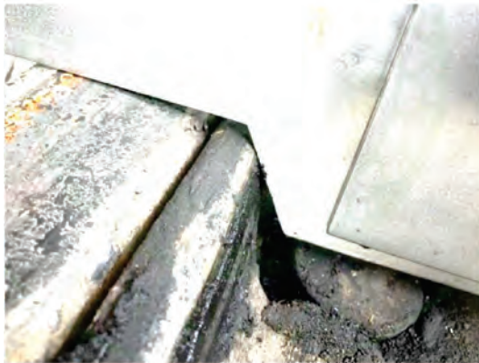
Gauge No.4, Switch No. 2, 20 in from the tongue's end, PASS or FAIL???
