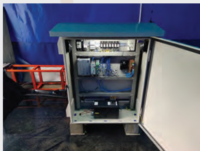
Water proof inspection
