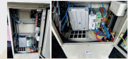
Water proof inspection
