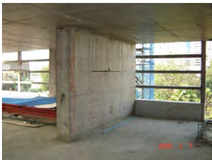
Addition of shear wall to RC building [1].
