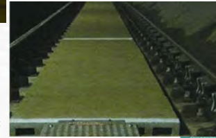
FIGURE 7-31 Absorptive treatment applied to slab track [7-16, 180 (18)].
