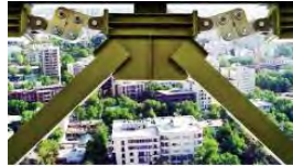
Yildirim et al. mentioned the rotational friction dampers to seismic retrofit of RC building. [4]
