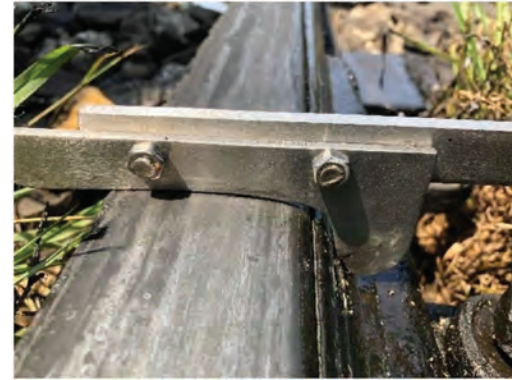
Gauge No.2, Switch No. 214, 10 in from the tongue's end Test at Bangsue Locomotive Depot
