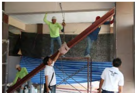
Addition of conventional brace to RC building [1].
