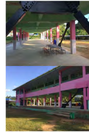
(a) Target 2-story bare RC school building (b) Retrofitted building with BRBs
