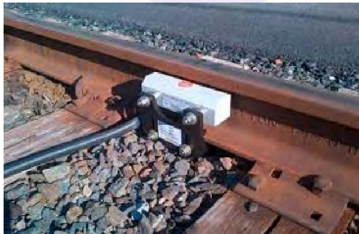
Example photograph of Loadcell installed on the rail.
